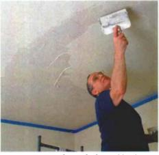
**Creating a seamless whole.** To blur the borders where different sections meet, new joint compound is lapped a few inches over the old (but still wet) mud.
