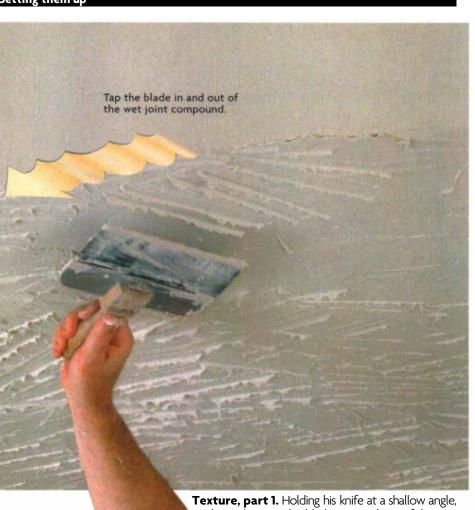
**Texture, part 1.** Holding his knife at a shallow angle, the author taps his blade into and out of the wet joint compound, making sharp ridges. To create a random appearance, he continually varies the direction of the strokes.
