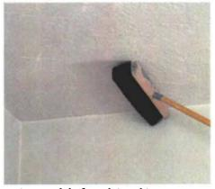
Wait a week before doing this. Scraping the wooden backside of a push broom over the dried texture knocks loose any fragile particles before they get caught in the paint roller.
